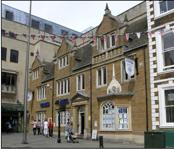
The Welsh House, Grade II Listed, is one of the buildings which the survived the fire.
