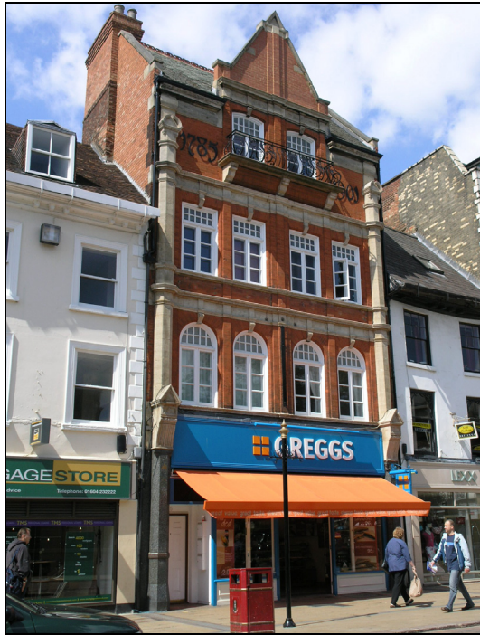
No. 5 Mercer's Row, 1901, is an imposing building along the street scene.
